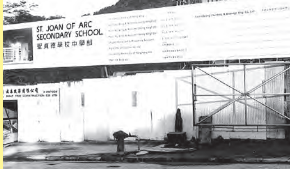
Our school campus under construction!
